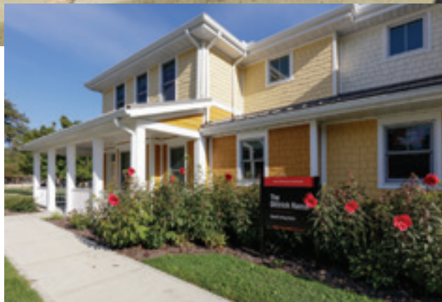
transformations included—east of Sandusky Street—the renovation of Merrick Hall, Edwards Gymnasium, and
